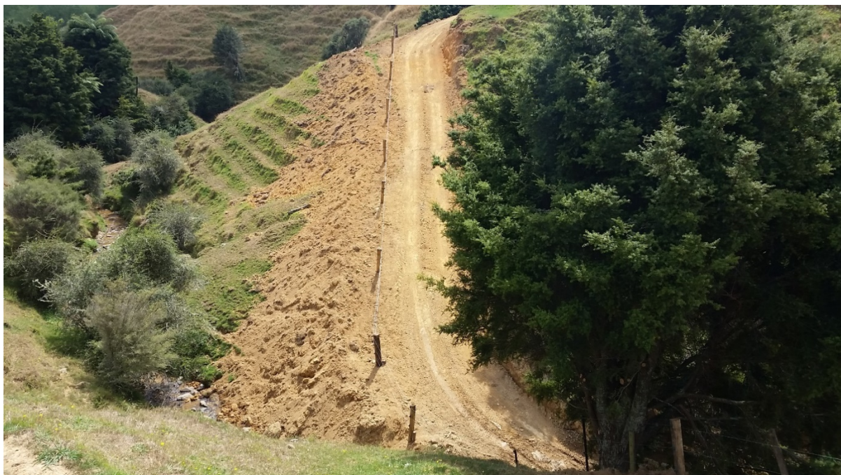
Figures 8 & 9: Bulldozed tracks for fence lines in hill country that are above streams
